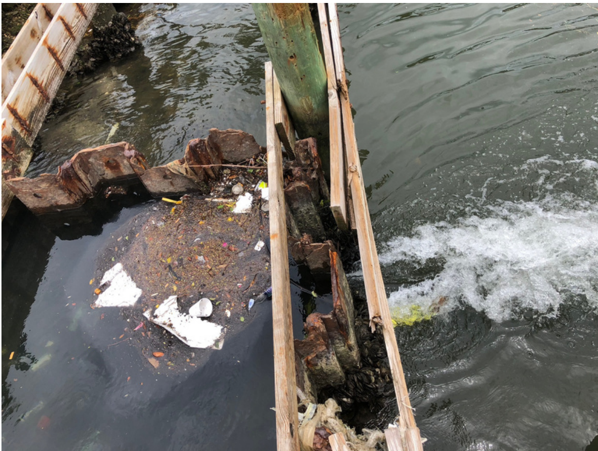
Figure 1. An outfall discharging stormwater in Coconut Grove.
